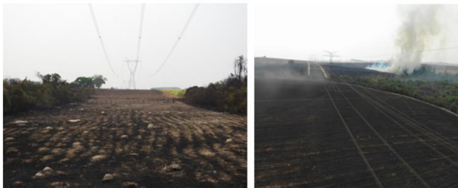
Figure. 11. Left: Wildfire under transmission line in the Ribeirão Preto Region (São Paulo State). Right: Fire near a transmission line in Bauru (São Paulo State) [Source: CTEEP].
