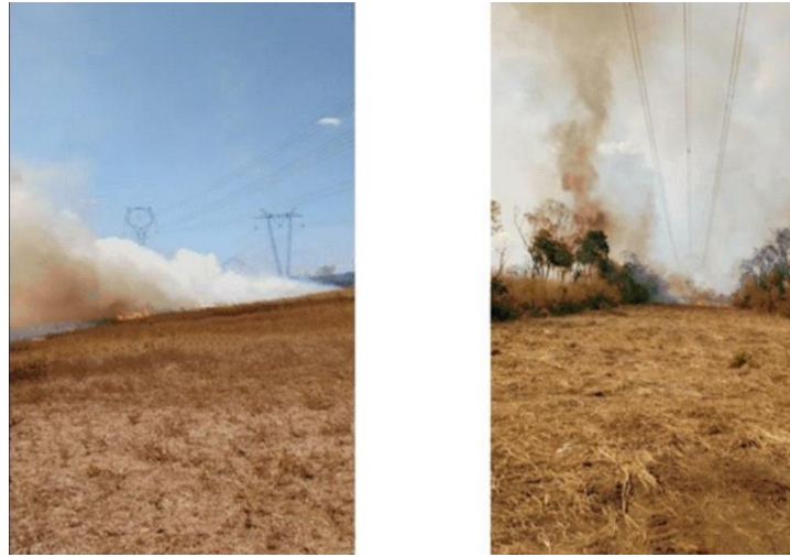
Figure. 12. Wildfires close to the transmission line in Tocantins [Source: National Electric System Operator].
